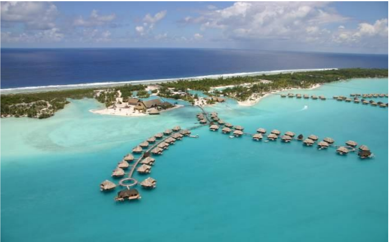
Bali Prefab project in Bora-Bora Tahiti (Four Seasons Hotel)
